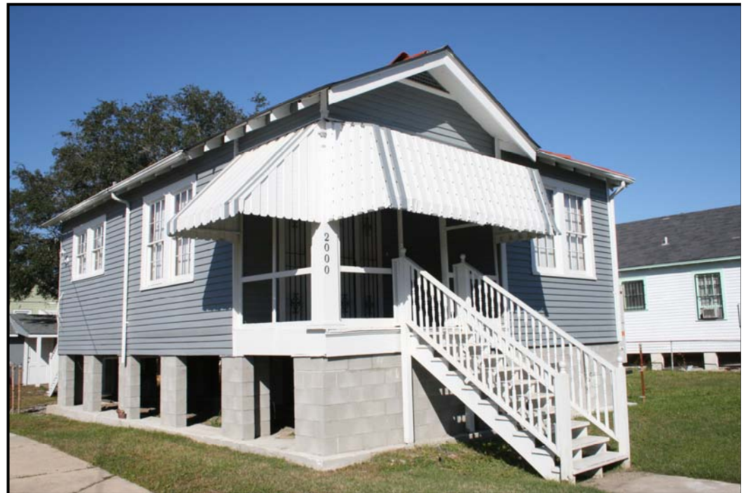
Elevated home in 9 th Ward
